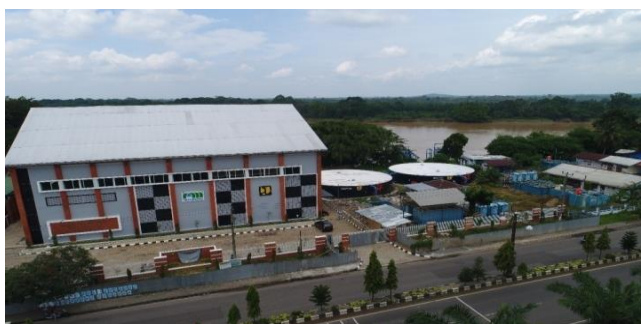
Gambar II-6 Water Treatment Plant (WTP) Kota Payakumbuh
